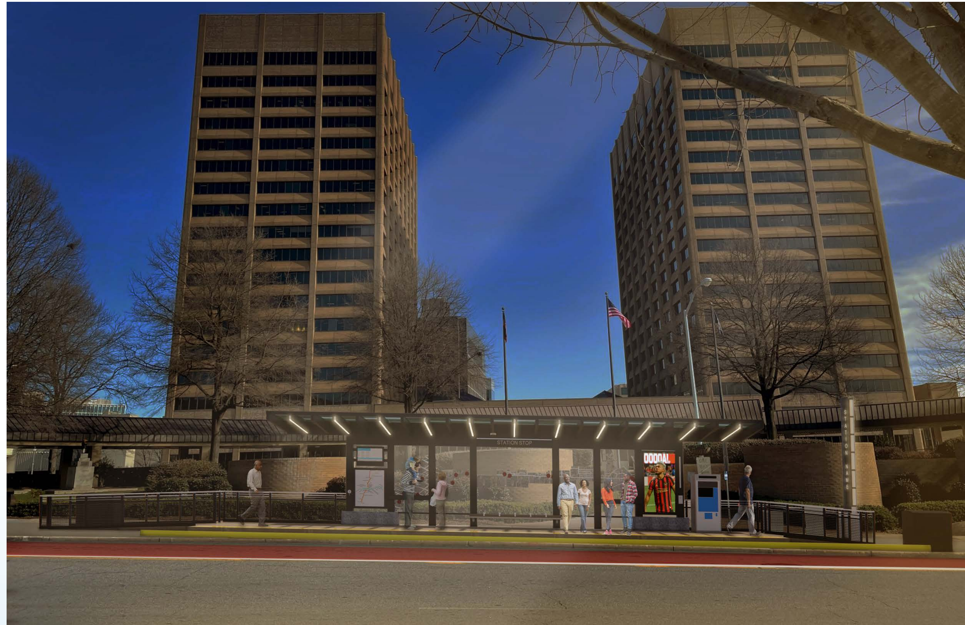
Georgia State Station Stop (looking north)
