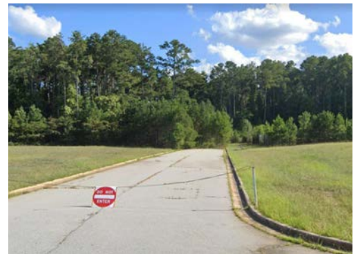
Stub roads on site
