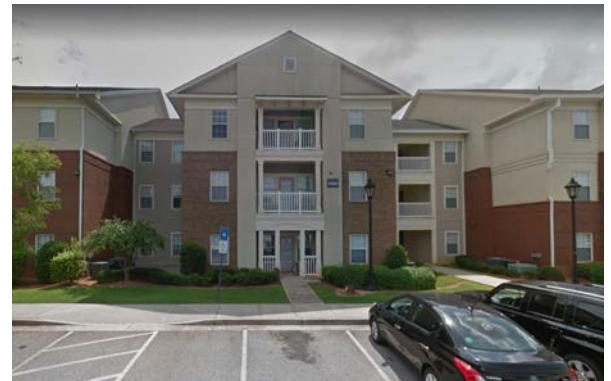
Existing multi-family housing
