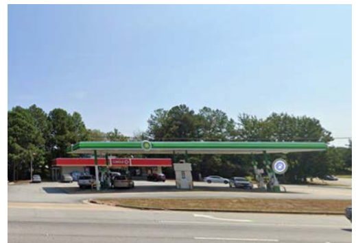
Existing gas station adjacent to site
