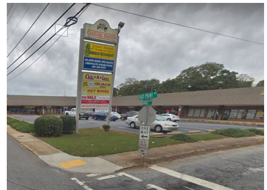
View from Northeast Corner
