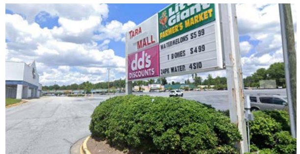
Aging signage, surface parking, and vacant retail spaces at Tara Crossings
