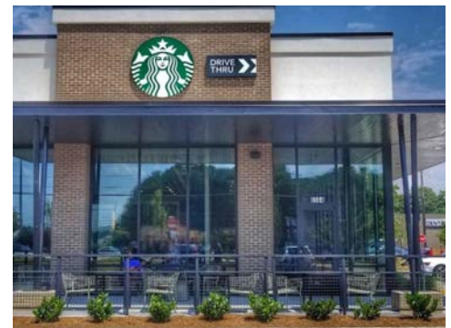
Existing, new Starbucks location
