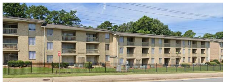
Aging multi-family buildings
