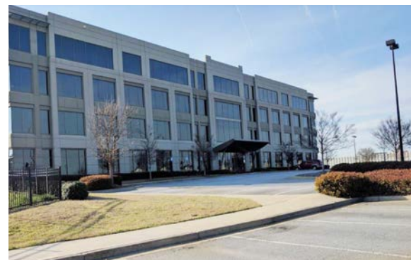
Existing office space in station area
