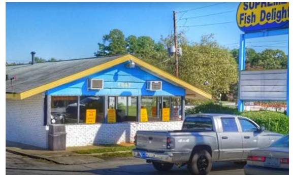
Stand-alone commercial building
