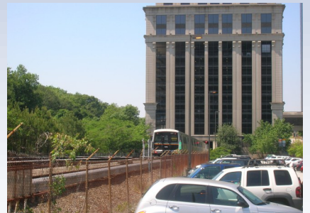
Resurgens Plaza Over MARTA Track Way
