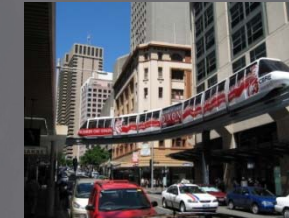
Automated Guideway Transit (AGT)
