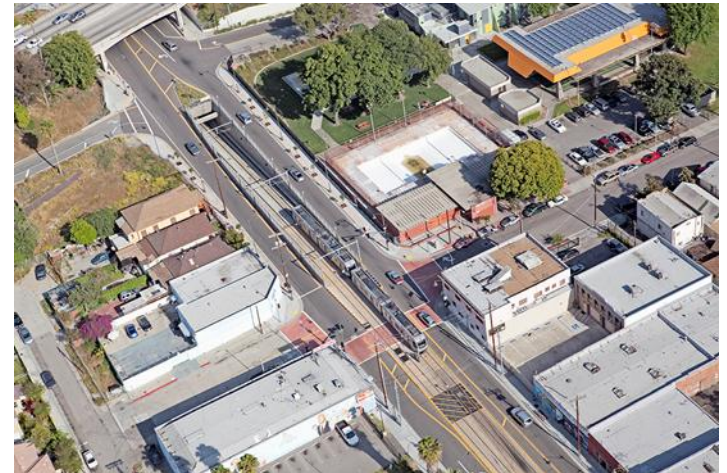
Transition from tunnel to street median (Los Angeles Gold Line)
