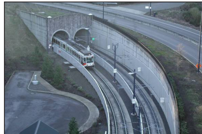
Example tunnel portal of MAX Light Rail, Portland, Oregon
